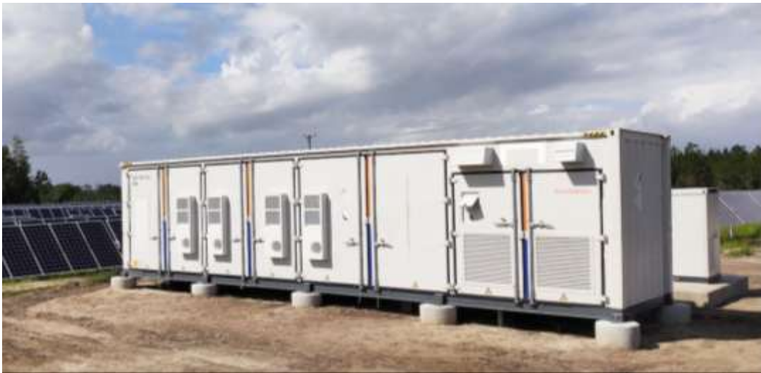
Figure 5.4 Typical BESS Container Example
